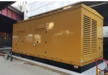
At Left: The station's new $1.3M generator will provide critical resiliency for passenger operations.
