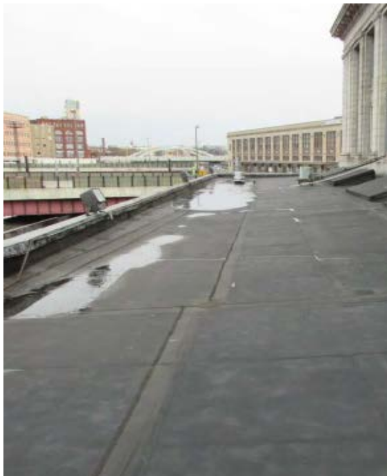
Station roof replacement under at nearly 100% design as part of SOGR program.
