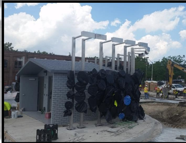
Operator Bathroom and Art Installation
